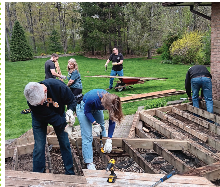
Joyce and Carl Heck's family works together to dismantle the porch.
